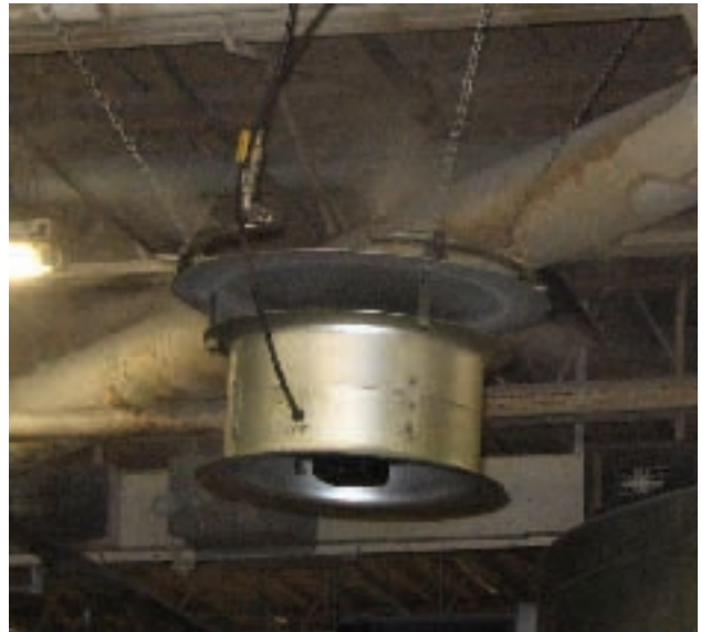
The Husson ML Princess unit (right) makes sure that stock doesn't lose water and begin changing dimensions
