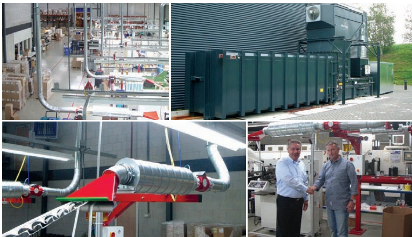
TOP LEFT: production environment with central pipe and a lot of EM-Modules (exhausting modules) for the extraction and cutting of edge trims and matrix TOP RIGHT: press container with air-material-separator, main ventilator and balance ventilator outside the plant. BOTTOM RIGHT: Josef Thor, Managing Director Matho GmbH; Right Jack Willemsz, Managing Director W&R etiketten shaking hands after finishing installation and acceptance of the system BOTTOM LEFT: EM-160 module on every label press, cuts the matrix and edge trim waste and extracts it through the main pipe to the press container outside.
